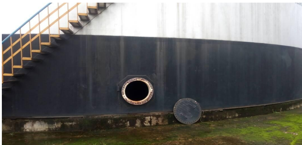
PLATE 5: The picture showing the effluent discharge point after washing the tank in Calabar jetty.
