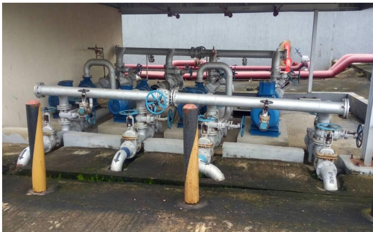
PLATE 3: The picture of the pump house, where products flow through from the tank farm to the gantry in Calabar jetty.
