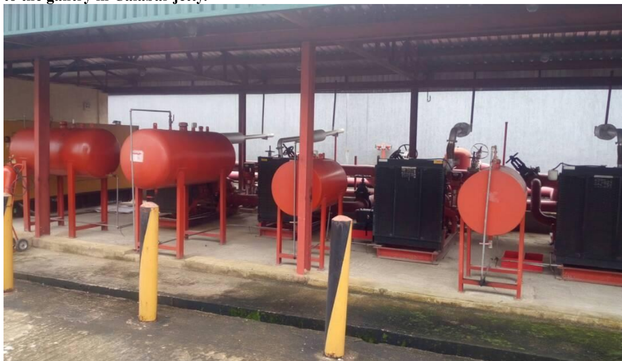
PLATE 4: Water and foam pumps used for washing the tanks in Calabar jetty.
